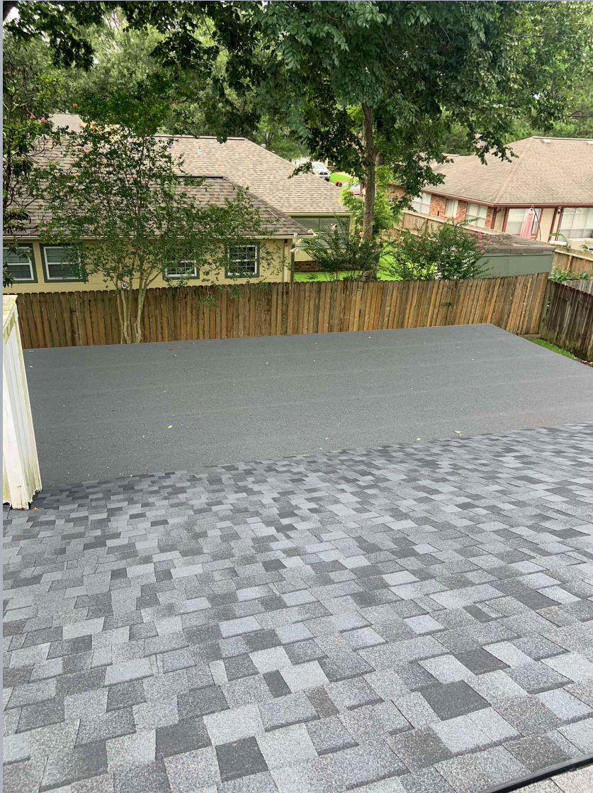
JDSI Roofing Picture Examples
