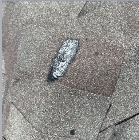
Finishing Corner Shingle
