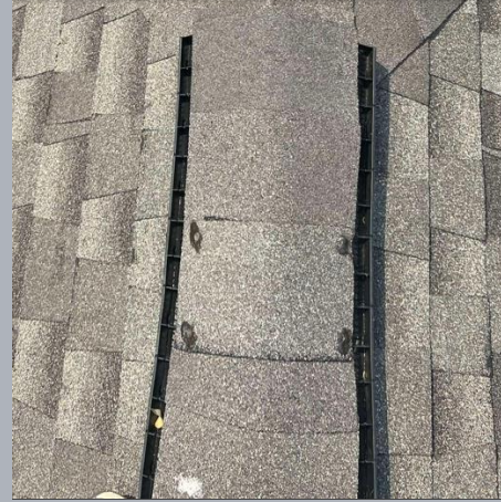
Finishing Cap Shingle
